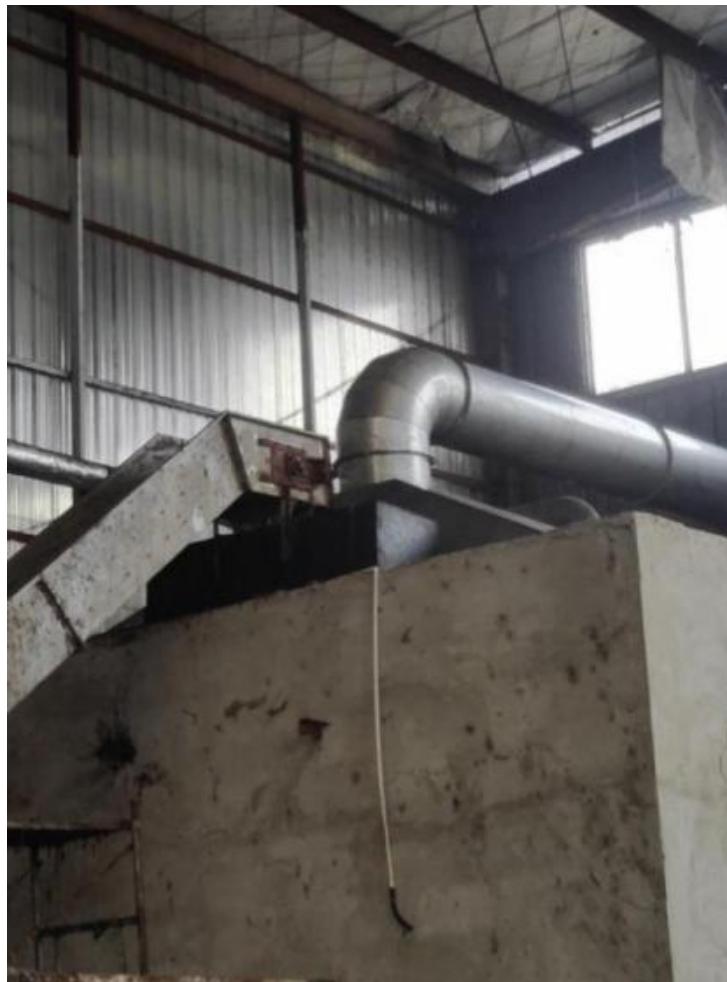
场内破碎系统加装集气罩
